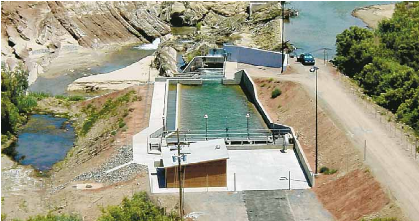
Overview of Diversion Dam and Fish Screens
