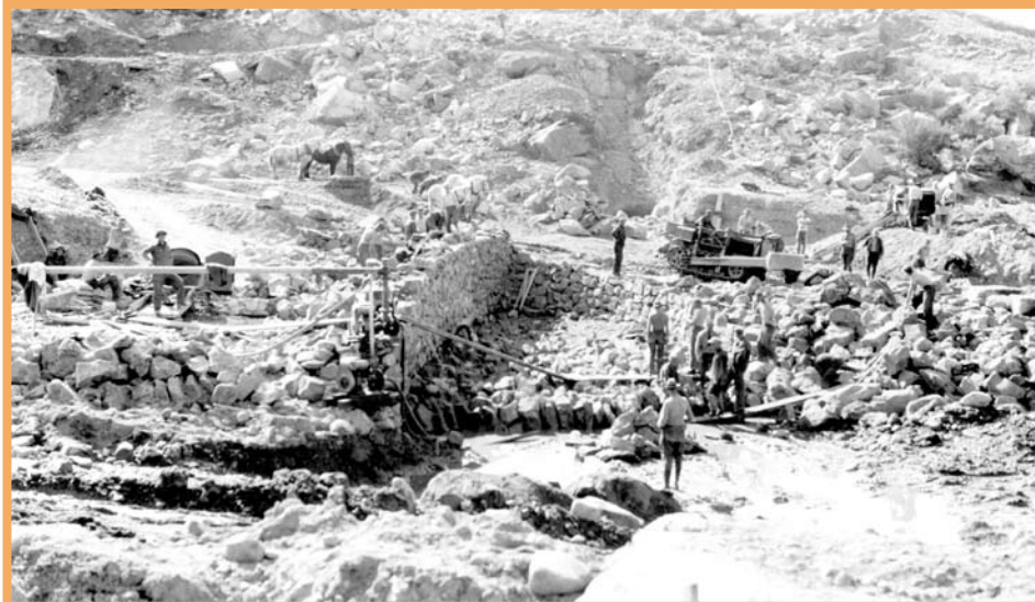
Excavation and beginning of south end of churning bowl — 1933
