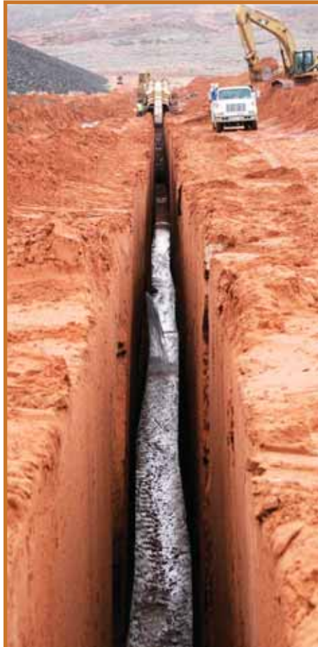
20-foot deep trench captures shallow groundwater of drinking water quality
